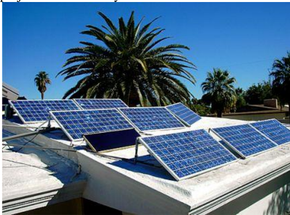
Fig: 6.9 solar panel of Bangladesh
